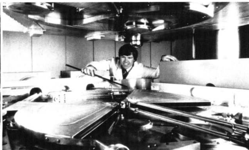
On April 13, 1985, two cyclotrons were delivered (Fig. 3) to the NIH Department of Nuclear Medicine, which had recently constructed a three-story underground facility to house them. Paul Plascjak, of the NIH cyclotron staff, checks the alignment of the cyclotron central region (Fig. 4). The ion source (long horizontal tubes in the lower right area) carries the gas to be ionized into the central region. The two delta-shaped objects are the dees that define the radiofrequency field. Directly in front of Mr. Plascjak is the water-cooled deflector, which extracts the beam on its largest orbit prior to exiting the cyclotron.
